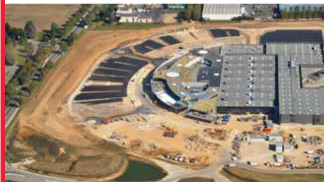
Centre commercial Leclerc - Barjouvillie (28)
