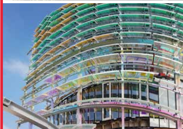
Hangar108 - Rouen Metropole (76)
