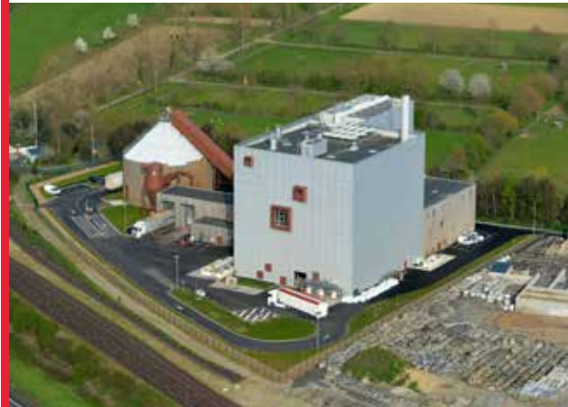
Dalkia CRE power station - Rennes (35)
