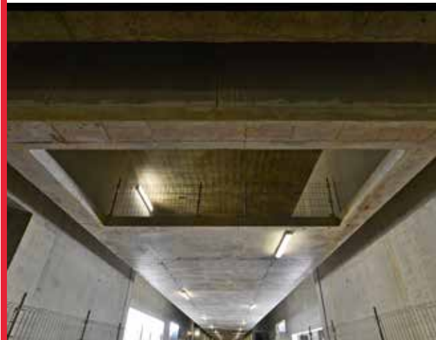
La Courrouze station - Metro Line B - Rennes (35)
