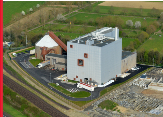
Dalkia CRE power station - Rennes (35)
