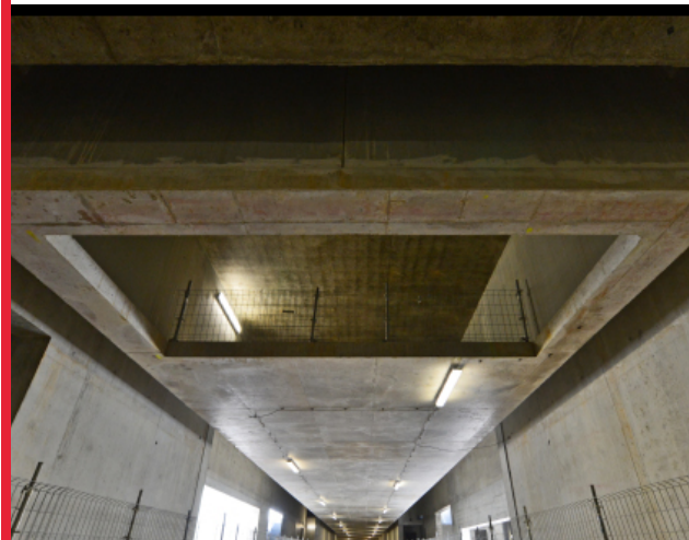
La Courrouze station - Metro Line B - Rennes (35)
